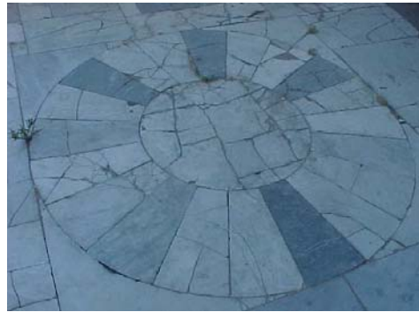
Marble Pavement in the Courtyard and in the Entrance
